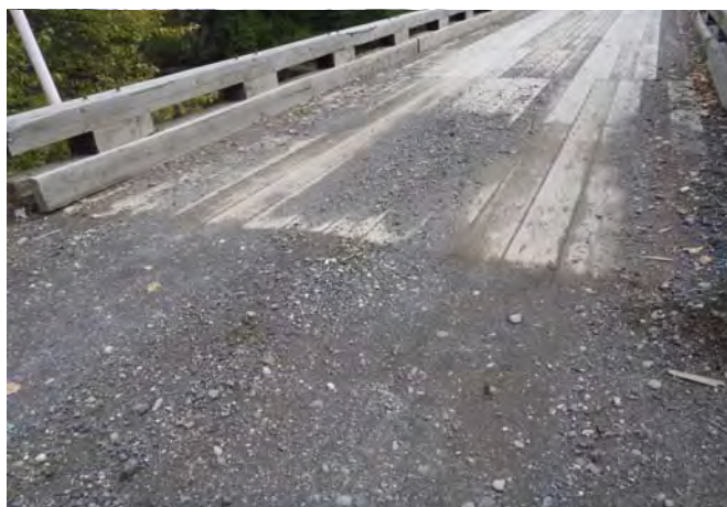
Figure 1-7: Camp end abutment joint.
