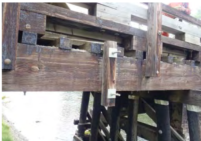
Figure 1-22: Span 3, stringer 9, downstream face.
