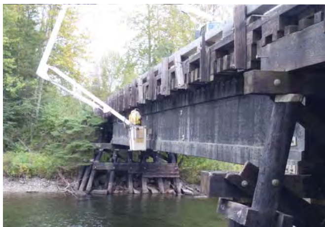
Figure 1-19: Span 2, girder 1, upstream face condition.
