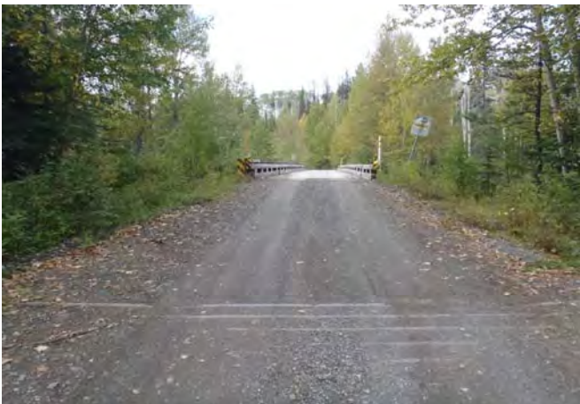
Figure 1-5: Looking towards camp end.
