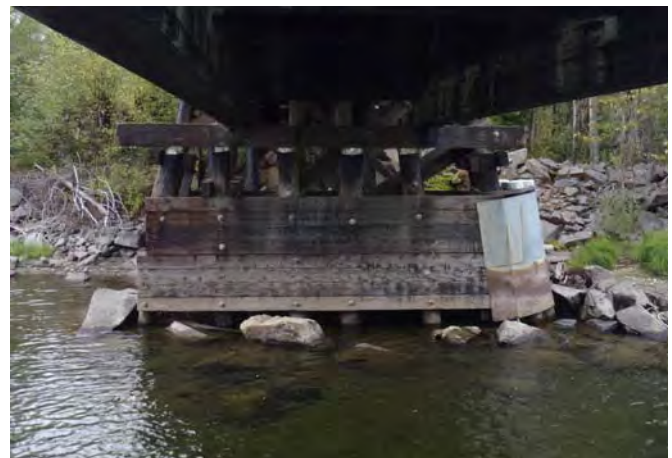
Figure 1-28: Pier 2, woods end face.
