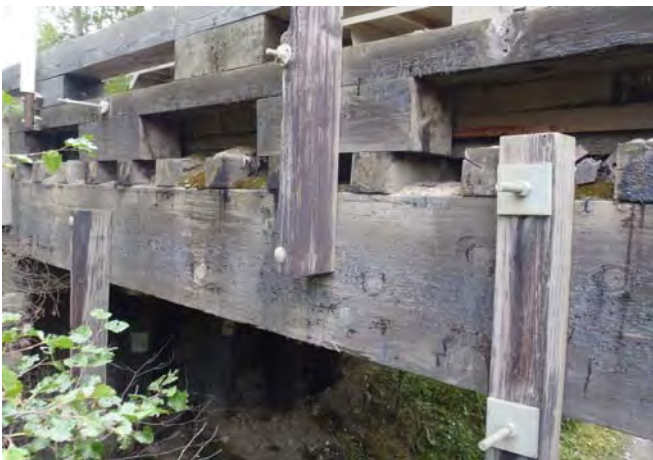
Figure 1-15: Span 1, stringer 1, upstream face.
