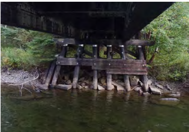
Figure 1-27: Pier 1 camp end face.
