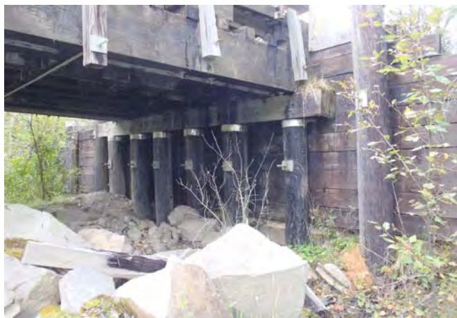
Figure 1-23: Camp end abutment.
