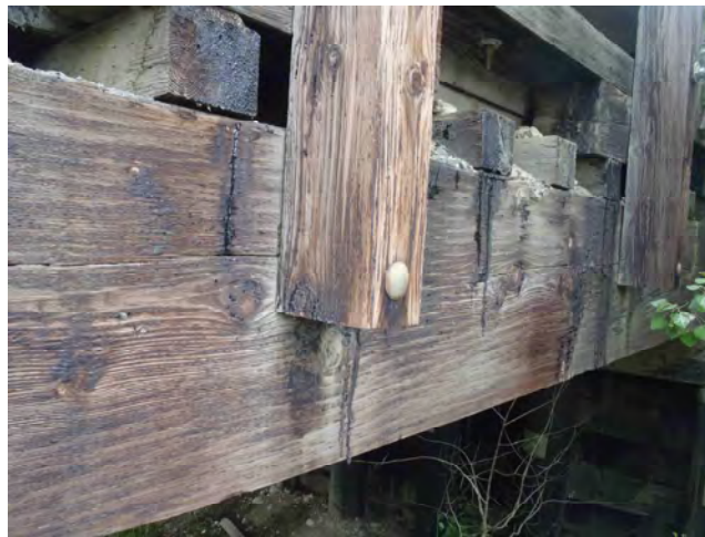
Example of Mid-Depth Series of Checks in Stringer, Span 1 Stringer 9 Downstream Face Shown
