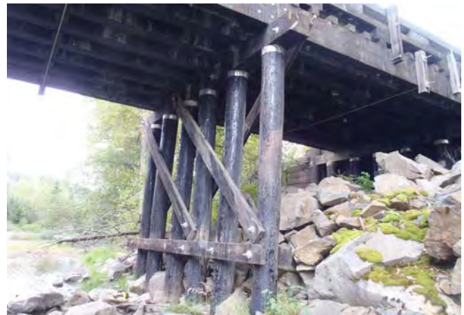
Figure 1-30: Pier 3, woods end face.
