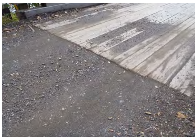
Figure 1-8: Woods end abutment joint.
