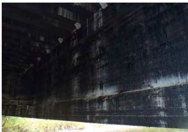
Figure 1-20: Span 2, typical interior girder face, girder 3 shown.
