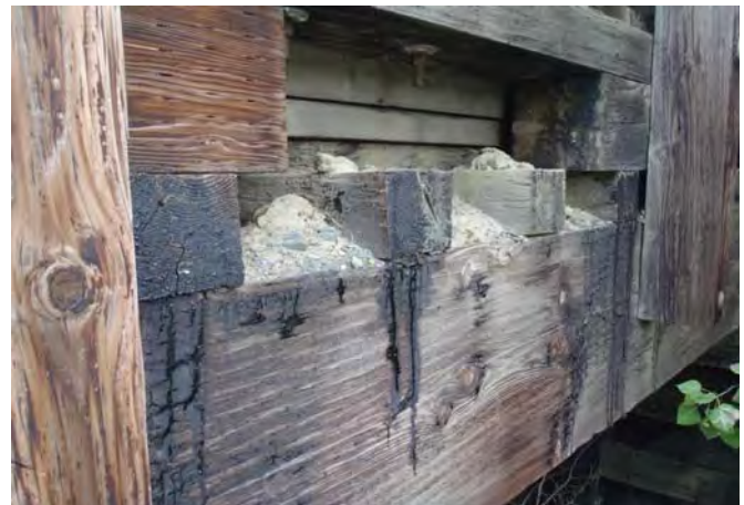
Figure 1-18: Span 1 stringer 9, downstream face condition, note debris accumulation.
