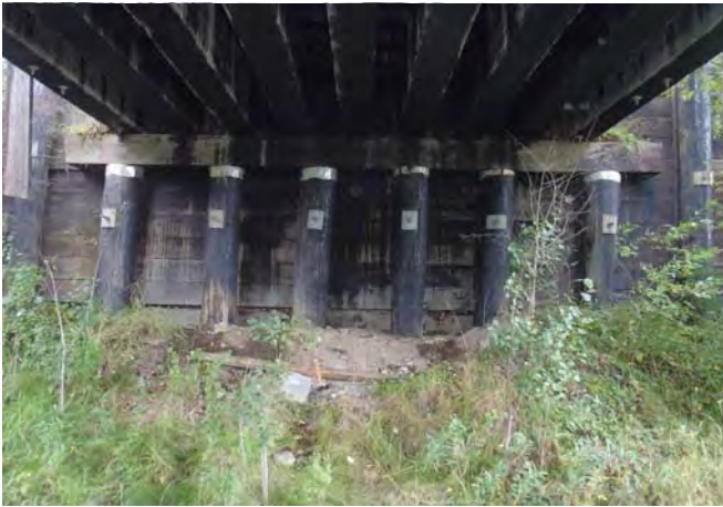
Figure 1-25: Woods end abutment.
