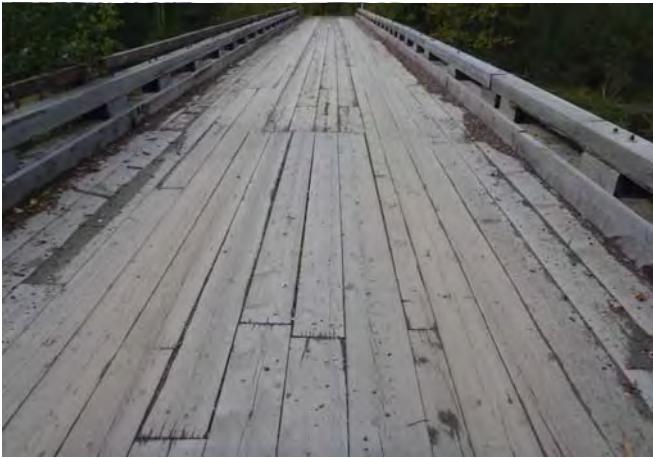
Figure 1-13: Typical deck condition.
